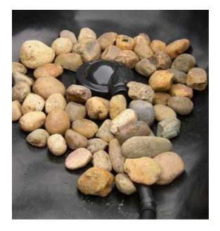
When installing an Aqua Art Retro-Drain, be sure to leave the area around the drain clear of rocks to allow free flow of water intake. Minimally:
