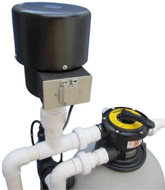
As shown in the picture: A blower is installed at the T of the inlet to the multiport valve. A ½ pound spring loaded check valve is installed below the blower and before the T. The flow direction is downward. The spring keeps the check valve closed at all time and is opened only when the blower is turned on, the pressure created by the air in the blower will force the check valve to open.
